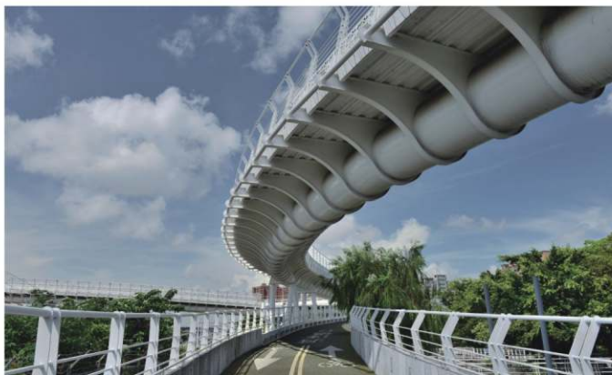
從翠華路自行車橋宛如龍骨的結構 Cueihua Road Bike Bridge's joist structure
