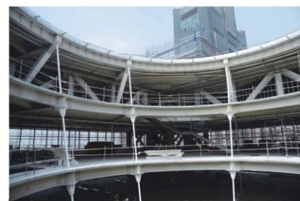
懸吊式結構 The suspended structural design
