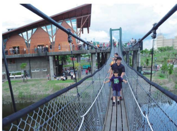
木棧吊橋 The wooden suspension bridges(Photo by Pao Chung-hui)
