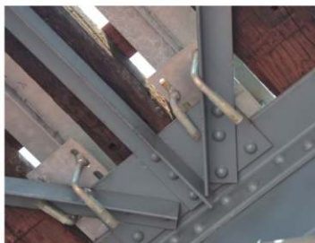
使用「夾具」方式固定於橋的本體 Clamps were used to fix the original structure.
