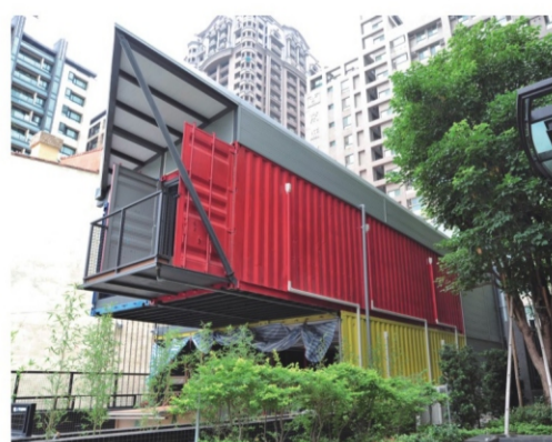
飛天糜鹿餐廳由貨櫃打造而成 Kaohsiung's Flyin' Moose Restaurant was built using cargo containers.
