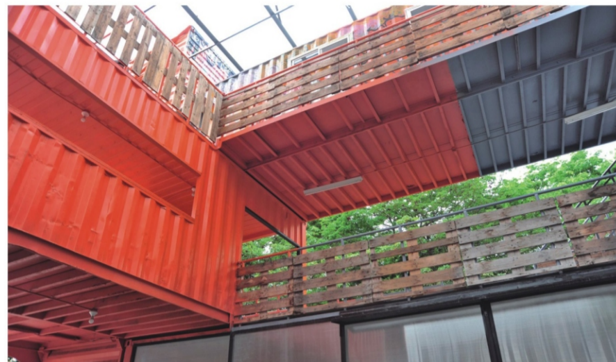
以13只貨櫃打造的貨櫃宅是高雄最大的貨櫃宅 Kaohsiung's largest cargo-container building has two stories and consists of 13 containers.
